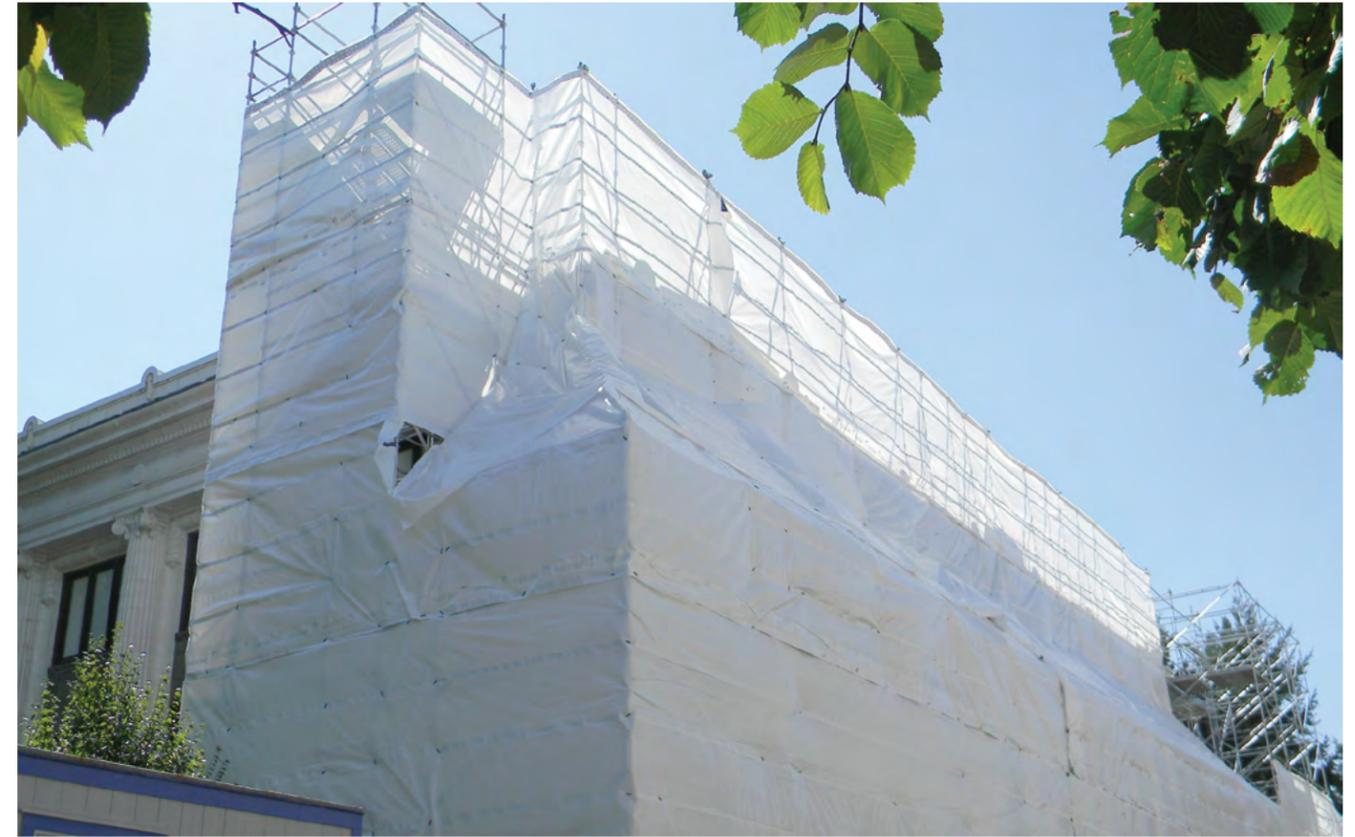
Supreme Court Building scaffolding on the north facade is draped with dust covering during rehabilitation work.
