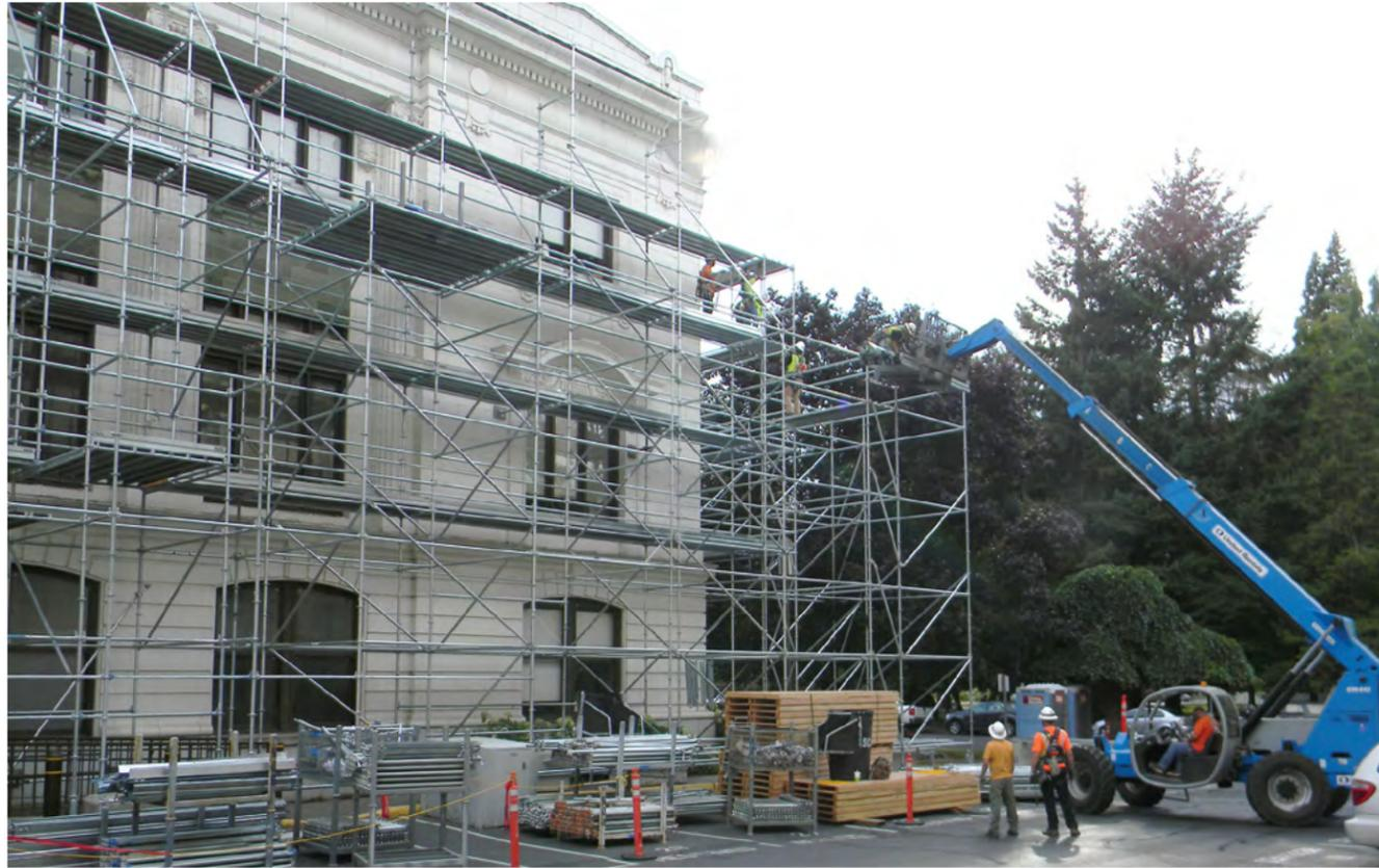
Workmen build scaffolding support system on the north facade of the Supreme Court Building, in preparation for rehabilitation work on the exterior of the building.
