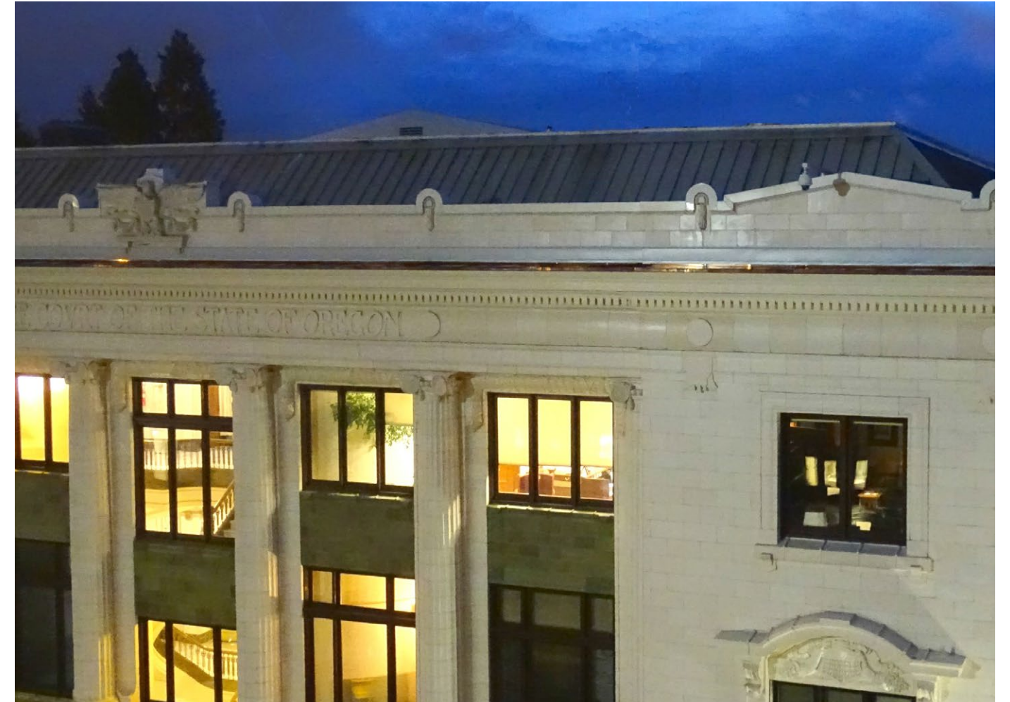
View of the interior of the Oregon Supreme Court Building alit in the evening.
