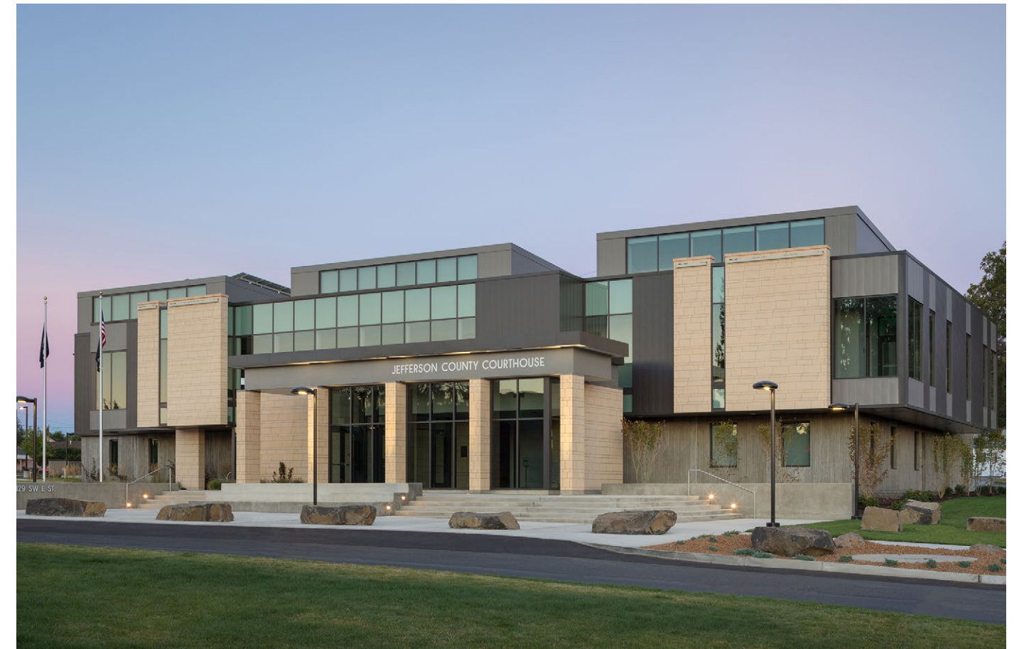
The new, completed Jefferson County Courthouse, exterior front view.
