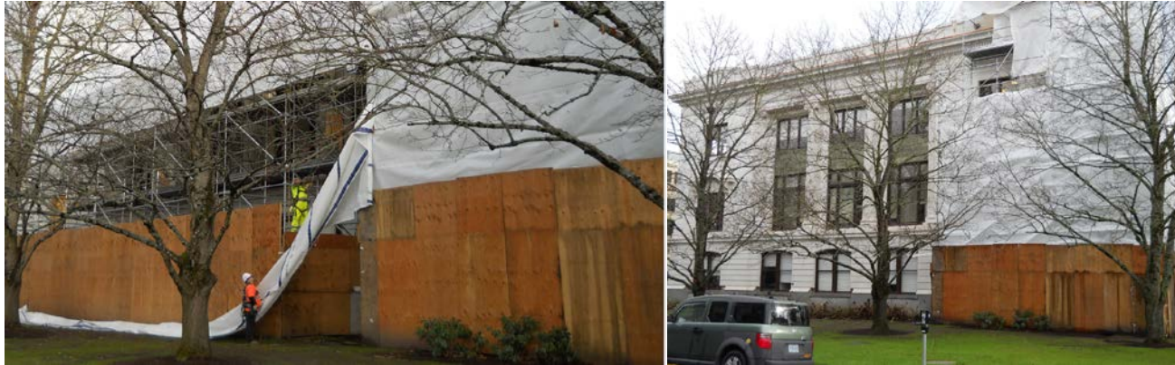
Scaffolding and protective cover for work
